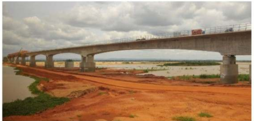
LOKO – OWETO BRIDGE, NASARAWA AND BENUE STATES (NORTH CENTRAL ZONE)
