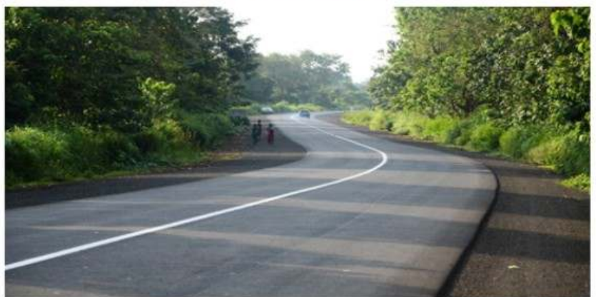
OTURKPO – OWETO HIGHWAY IN BENUE STATE (SECTION 1)
