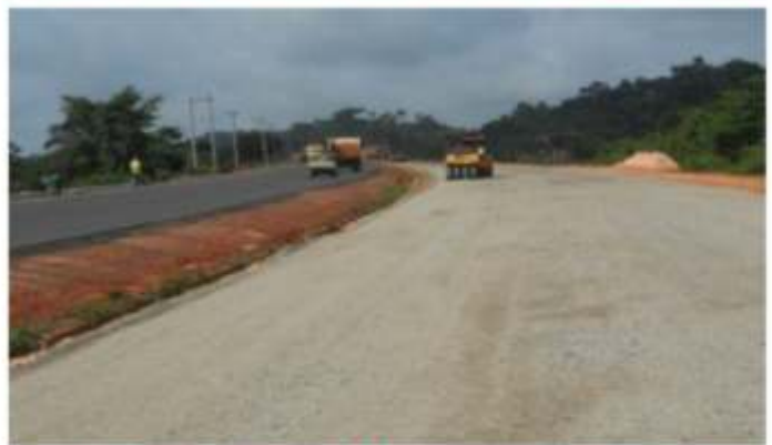
ENUGU – PORT HARCOURT HIGHWAY
