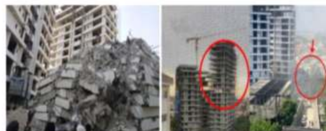
Figure 6: (a) Collapse of 21-storey Apartment Block in Ikoyi-Lagos, and (b) Other Structures
