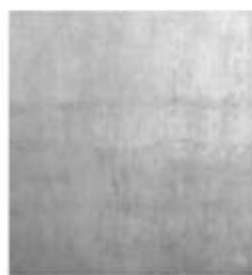
Figure 1 (b): Finished Concrete Surface
