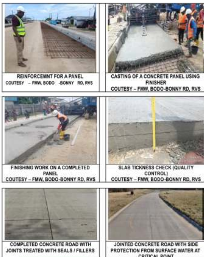
FIGURE 4: JOINTED REINFORCED CONCRETE ROAD CONSTRUCTION
