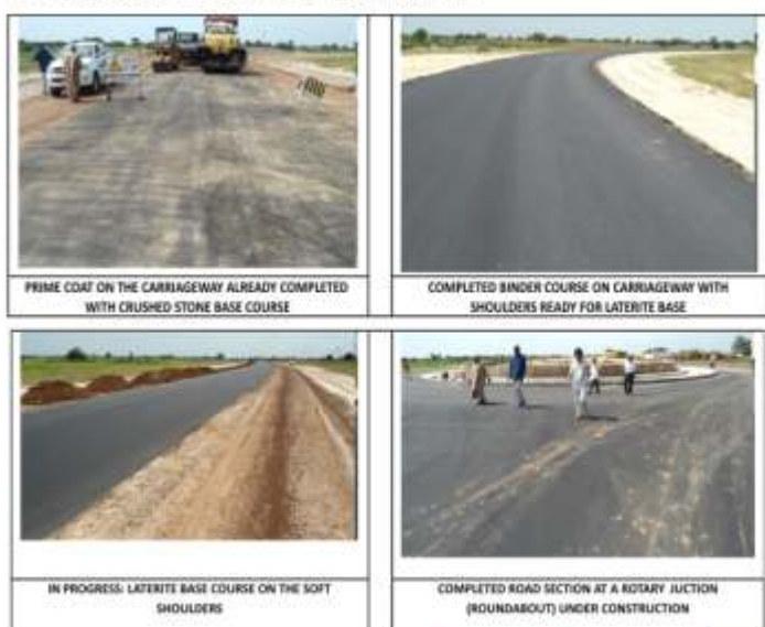
FIGURE 5: THE PROJECT'S PICTORIAL PROGRESS / ACHIEVEMENTS 3
