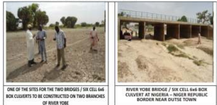
FIGURE 4: SITE OF A PROPOSED BRIDGE AND THE EXISTING SIMILAR ONE 2,3
